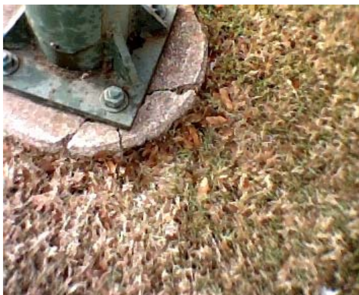
FIGURE 7 Cracked foundation.
